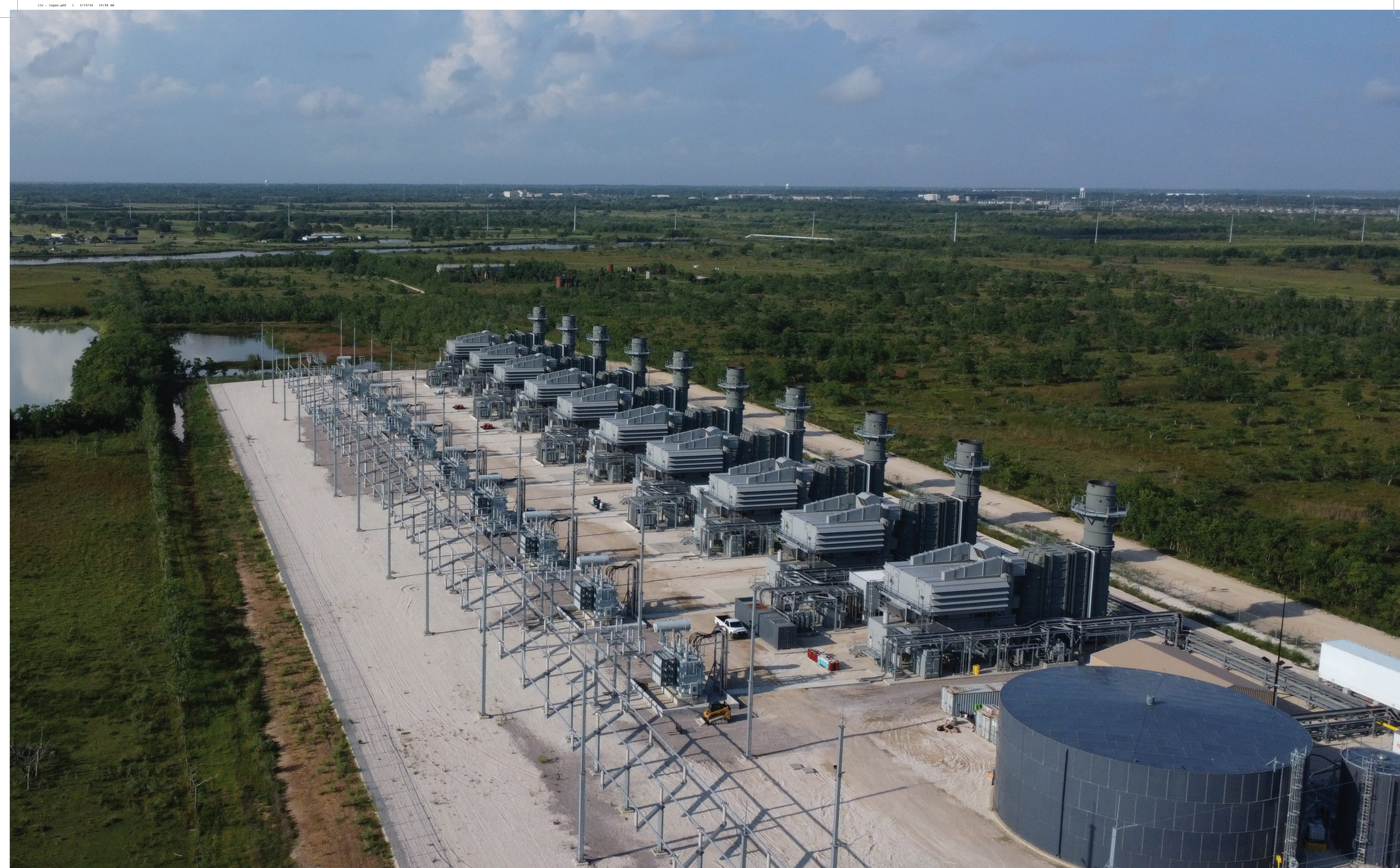
Topaz Generating Station near Houston, Texas / Centrale électrique Topaz près de Houston, Texas
